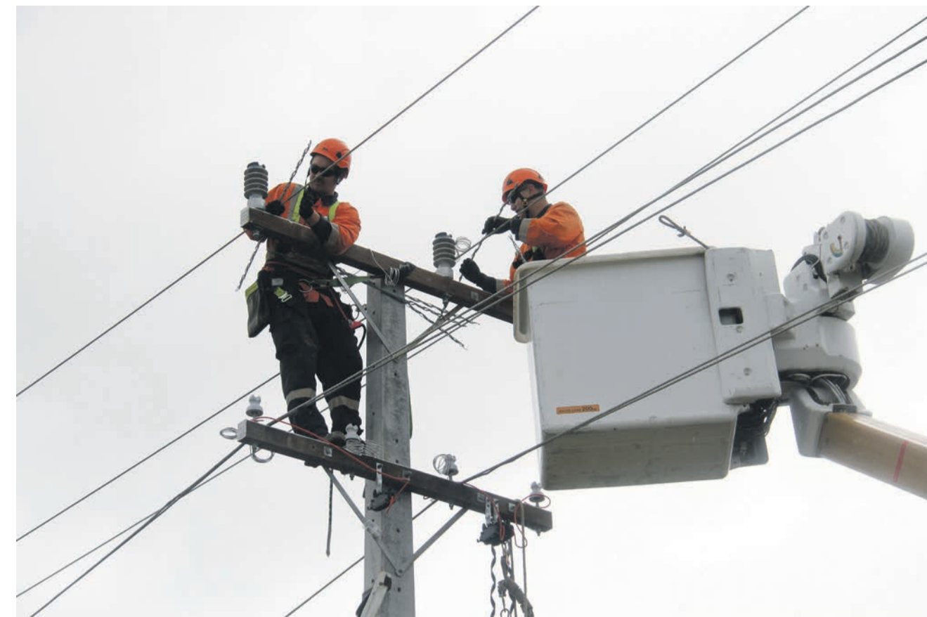
Powerco staff replacing poles at Oeo.
